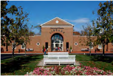
The New Albany Branch is the CML facility closest to the overall square footage per capita recommendation, at 1.0 SF/Capita for its current population.
