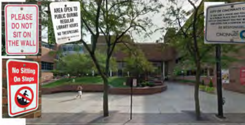
The Vine Street entry with elevated plaza has been a source of persistent complaints. Using this entry is tantamount to running a gauntlet. See the Recommendations section for proposed improvements.
