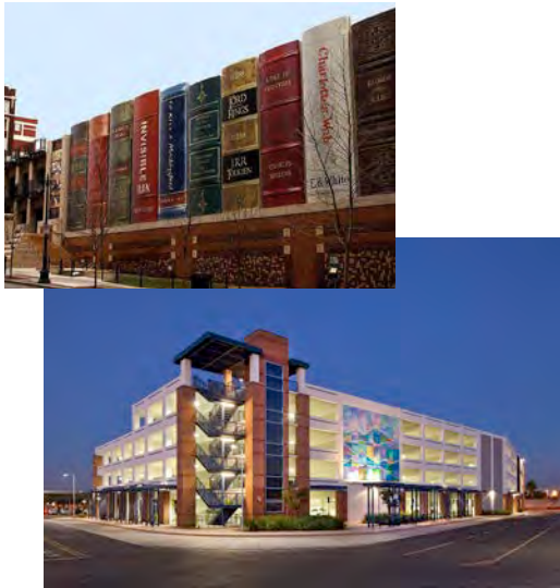
The Central Library parking garage at Kansas City Public Library (MO) features retail on the ground floor and four tiers of parking for library visitors.
