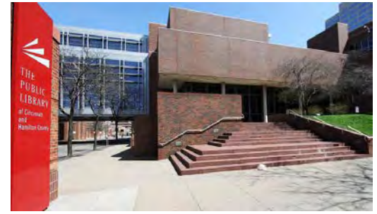
The multi-level plaza on Vine Street hinders accessibility to the Main Library.
