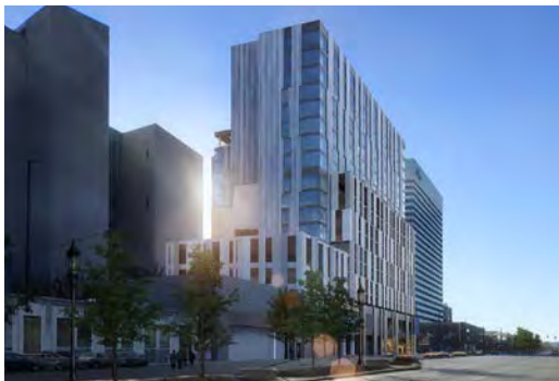
The "Kroger Development" is a major new mixed-use project just around the corner from the Main Library.
