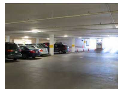
Basement parking garage
