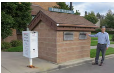
The Neighborhood Libraries (opposite) are equipped with basic library services for customers living in the immediate vicinity
