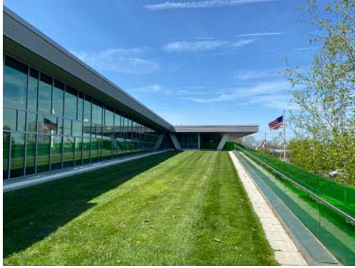
Living roof at the Parma-Snow Branch Library
