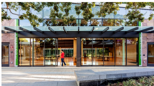
An example of a retractable door connecting a community room to an outdoor terrace.
